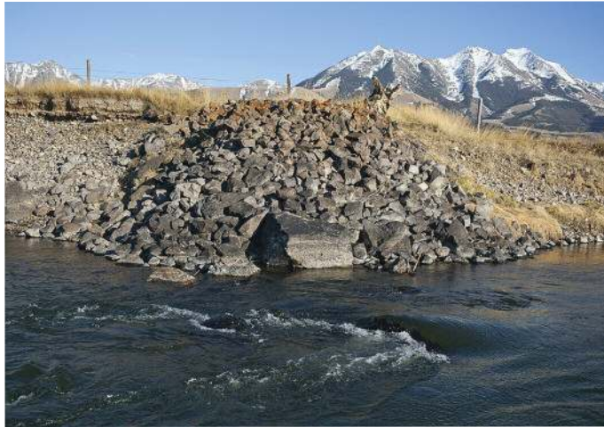
Riprap dumped along the riverbank.
