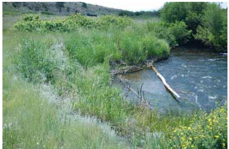
Using a biodegradable erosion stream blanket and locally harvested willow fascine (living branches bound together in long tubular bundles) to decrease flow velocity near the banks, erosion is being controlled after one growing season.
