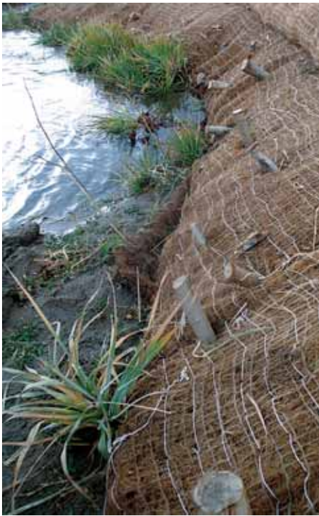
This erosion-control blanket of coconut fiber and cotton string is completely biodegradable. Dormant wood stakes are used to anchor it.
