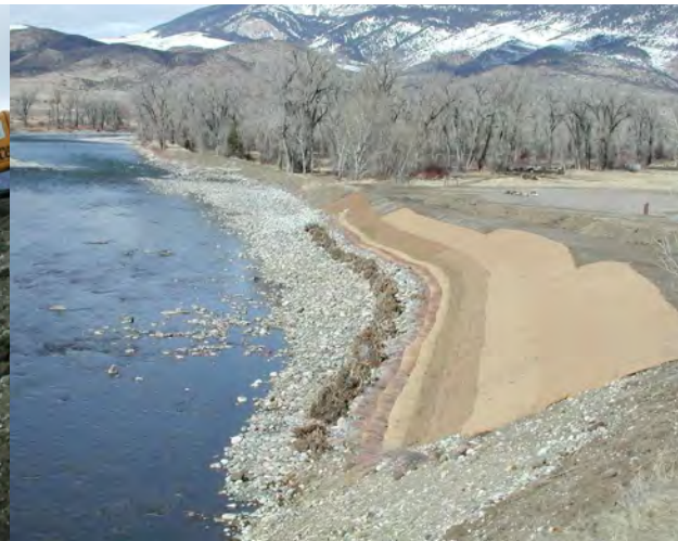
Erosion treatment complete
