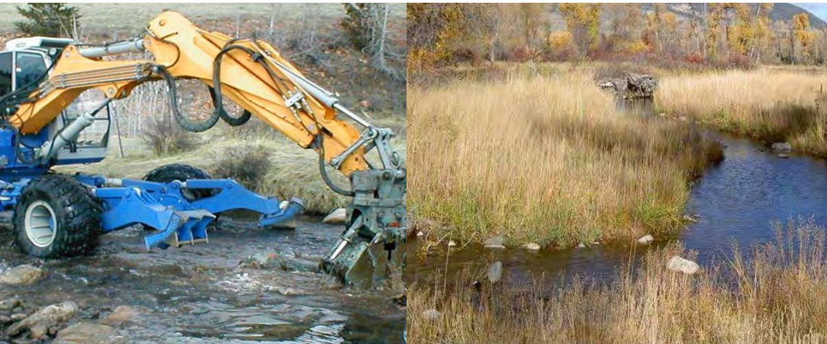
Constructed wetland first season
