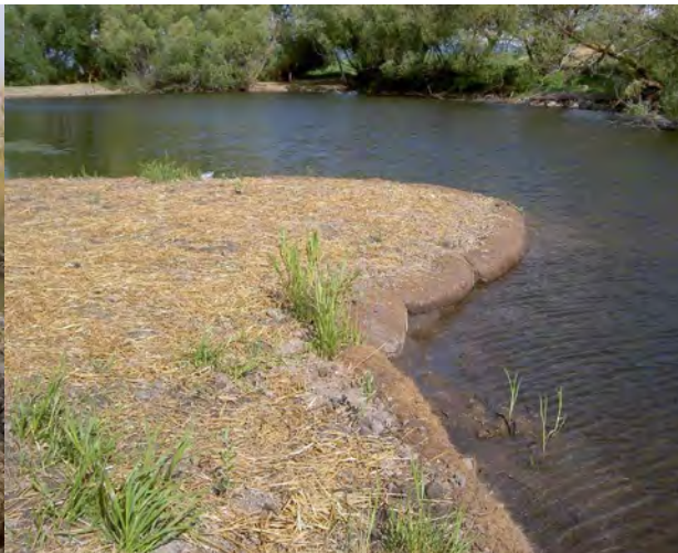
Detail of biostabilization along shoreline
