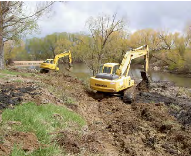
Wetland enhancement construction
