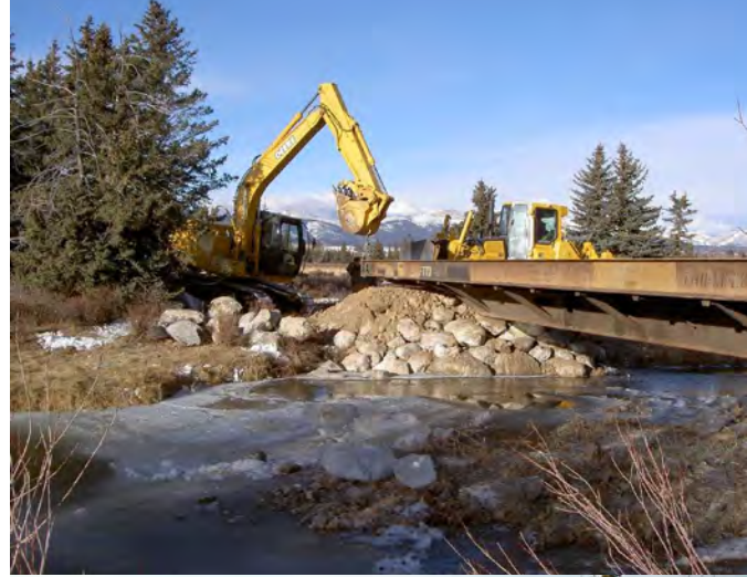
Property access bridge constructed
