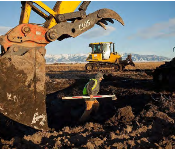
New channel construction
