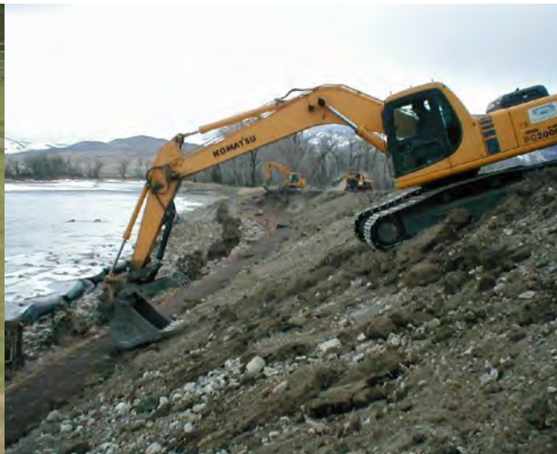
Mixed construction uses stone, vegetation and reinforcement materials
