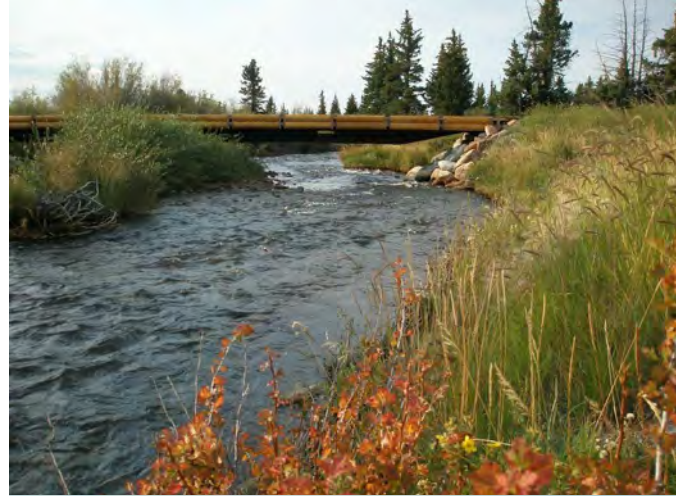
Restored streambanks and bridge site
