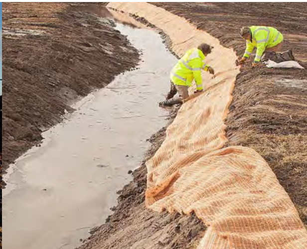
Erosion control materials added to banks
