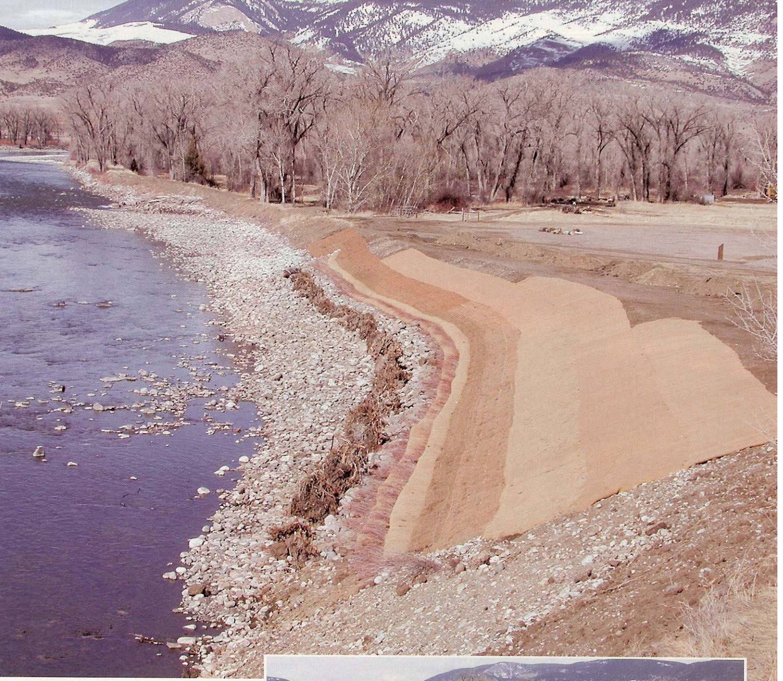
ABOVE: C125 double-net, 100% coconut fiber blankets were installed on the upper slope. These slow-degrading fiber and stabilized nettings blankets provide up to 36 months of protection for slopes exceeding 1:1.
