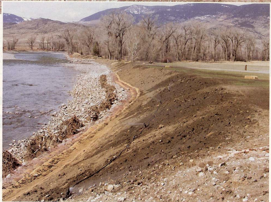
ABOVE: C125 double-net, 100% coconut fiber blankets were installed on the upper slope. These slow-degrading fiber and stabilized nettings blankets provide up to 36 months of protection for slopes exceeding 1:1.
